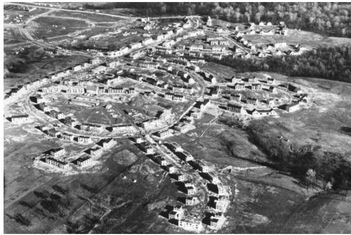
Greenhills, Ohio under construction in the 1930s
